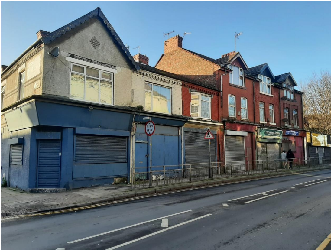
Linacre Road at the junction with Lily Road
